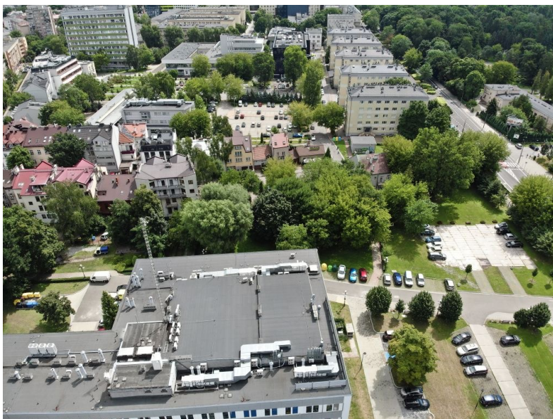
The site surroundings. The mast is mounted on a rooftop of the building in the bottom left corner.
